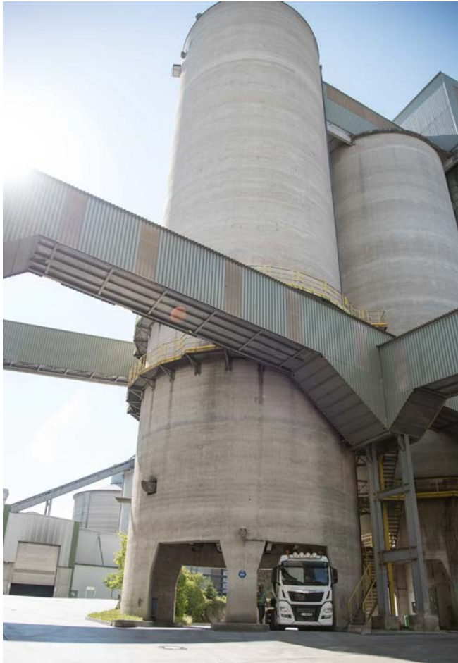
Automated loading at cement silo.
